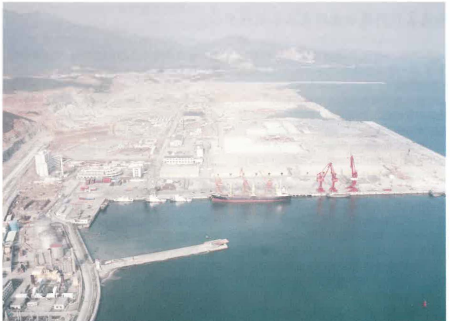
Another shot from the air with cranes being erected.
